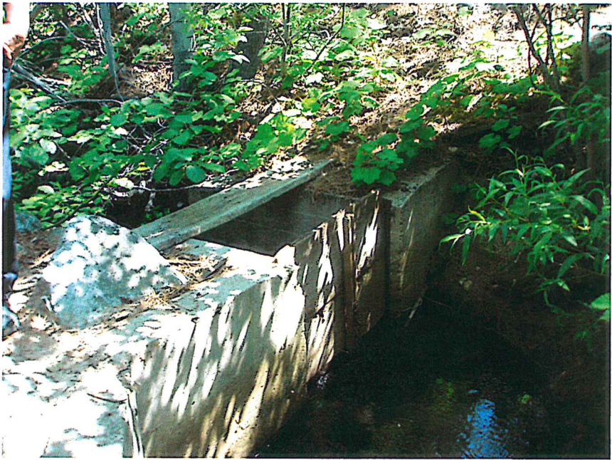
View of irrigation diversion structure.
