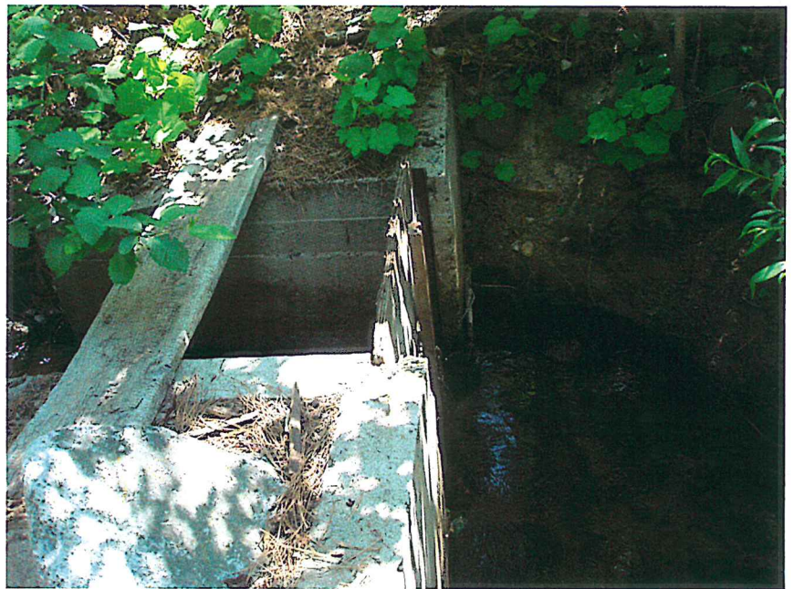
View of irrigation diversion structure.
