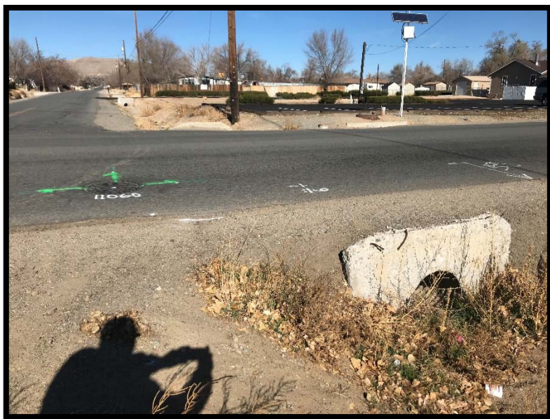
Figure 8 – Culvert crossing E. 4 th Avenue
