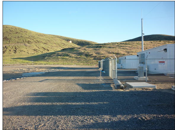
PHOTO 2: SOUTHWEST CORNER LOOKING NORTH.
