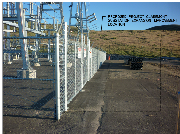
PHOTO 4: SOUTHEAST CORNER LOOKING NORTH.
