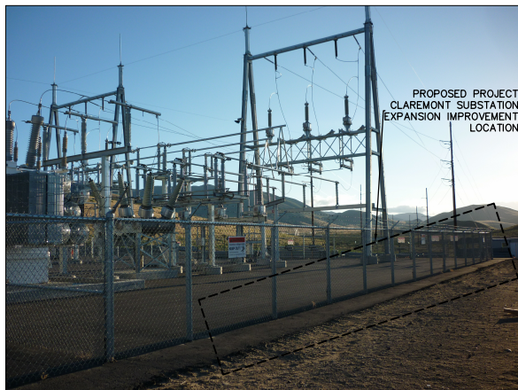
PHOTO 3: SOUTHWEST CORNER LOOKING EAST.
