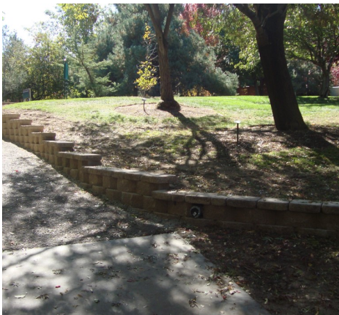
New Retaining wall at Evans Creek Bridge
