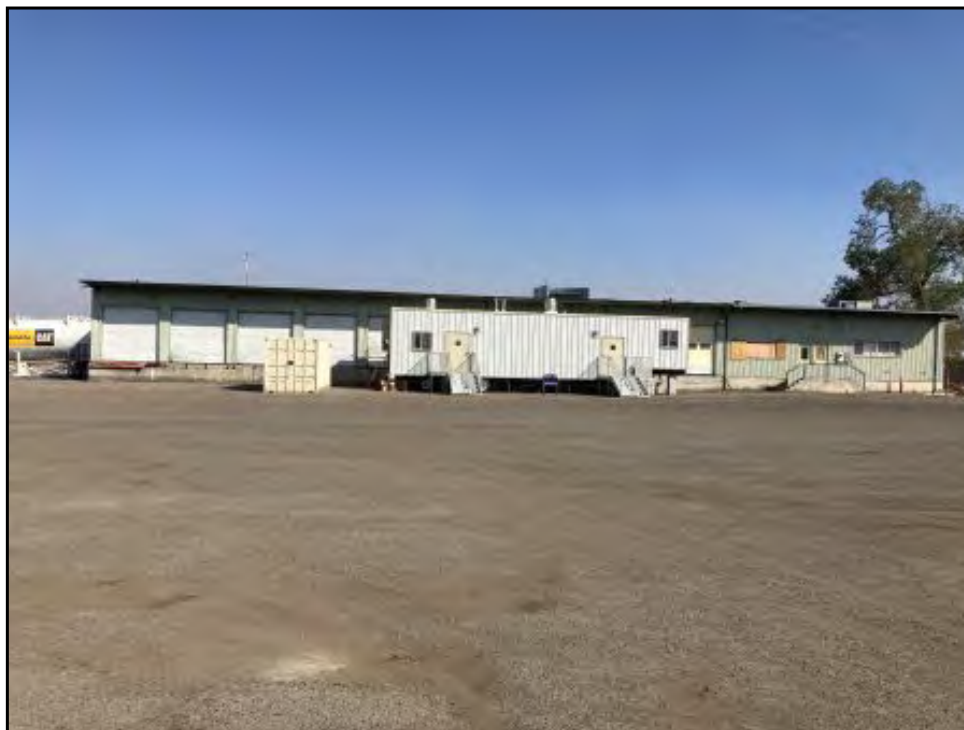
19 : View of the Subject Property transit warehouse building exterior.
