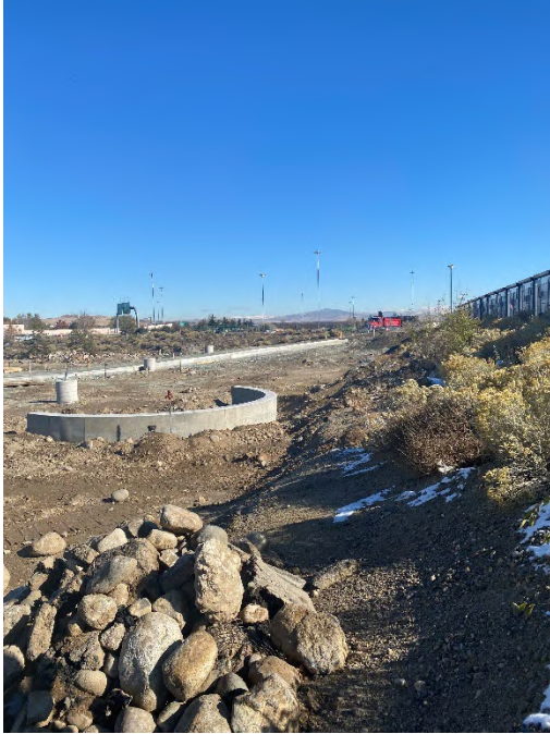
Photo 17 View to the northeast along the southern Site boundary (November 2022).
