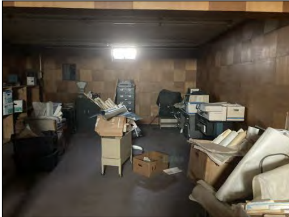
5 : View of the Subject Property office building basement interior.
