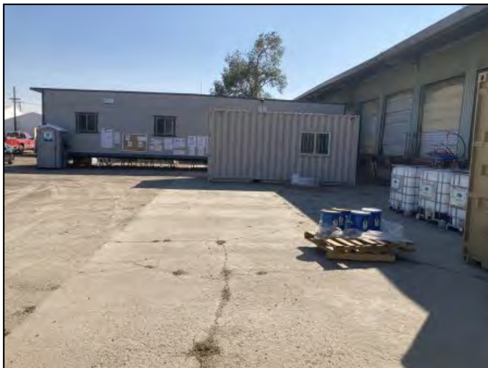
20 : View of the Subject Property transit warehouse building exterior.
