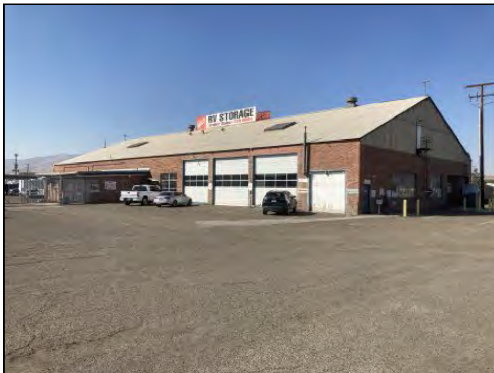
7 : View of the Subject Property service garage building exterior.
