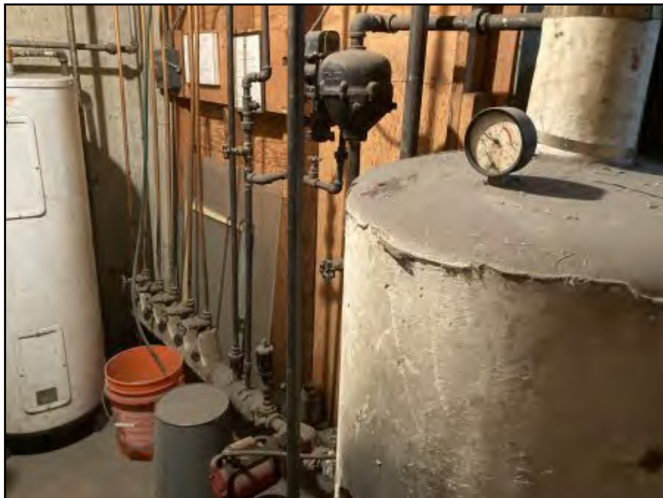
6 : View of the Subject Property office building basement interior.
