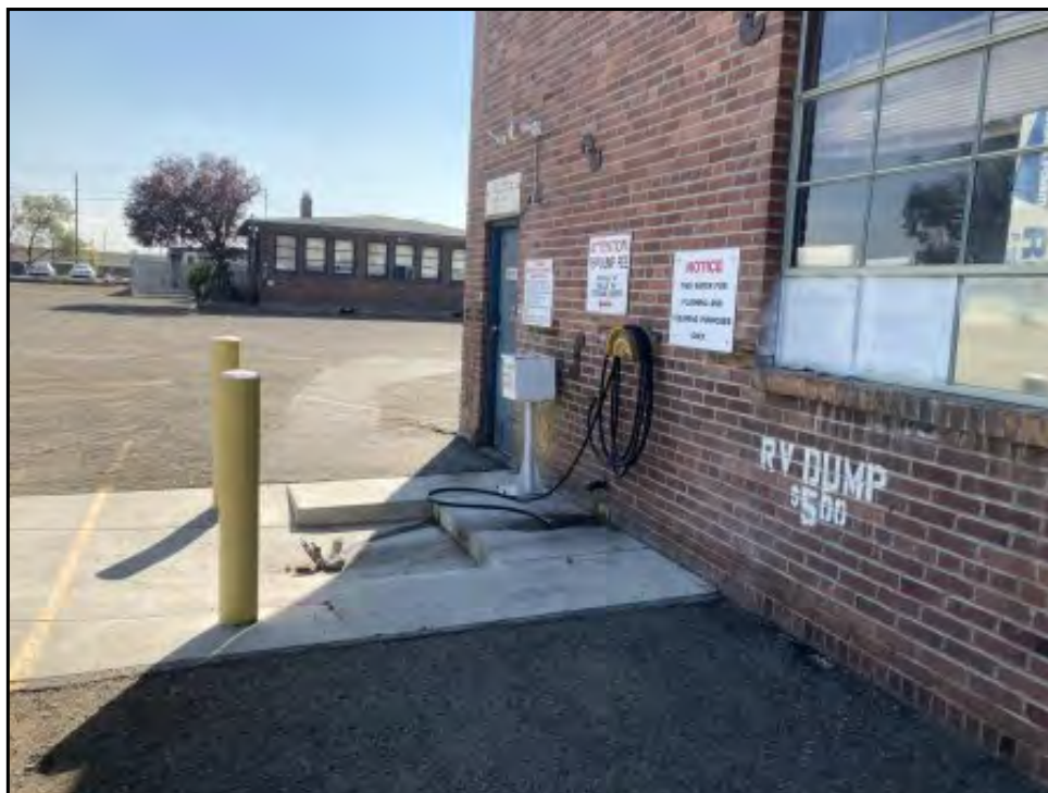
28 : View of the central portion of the Subject Property, looking south - including RV dump station.
