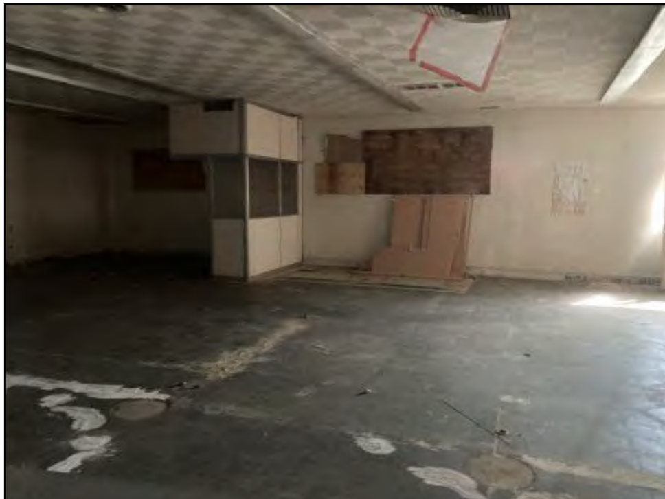
22 : View of the Subject Property transit warehouse building interior.
