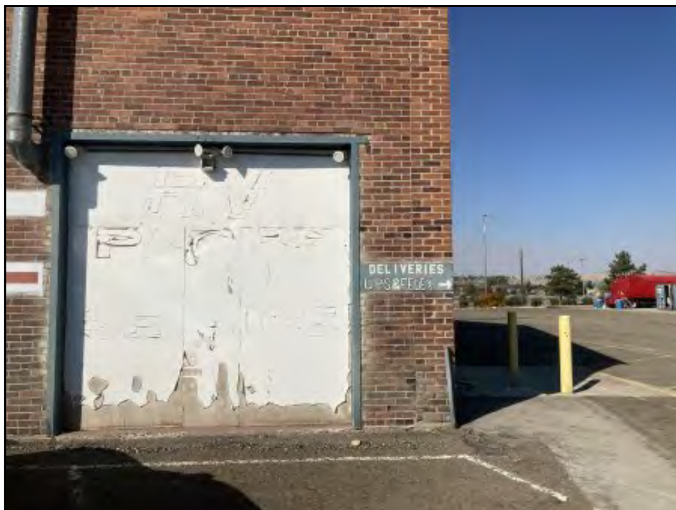
8 : View of the Subject Property service garage building exterior.
