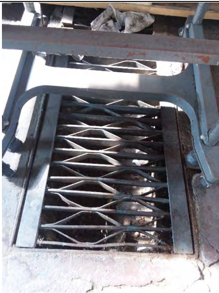
11. Floor drain in mechanics garage
