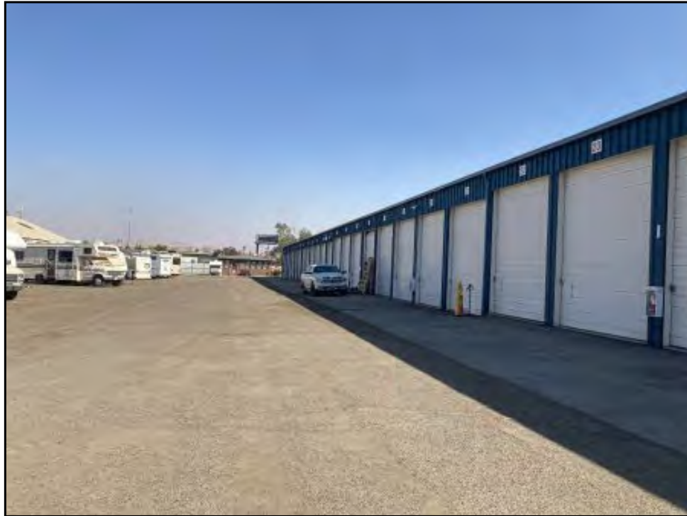
23 : View of the Subject Property storage warehouse building exterior.
