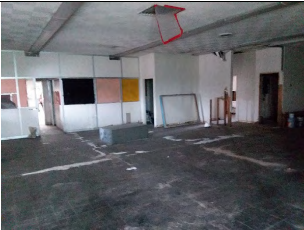
15. Office space of trucking transfer building
