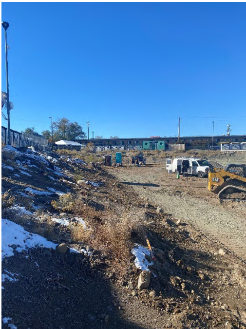
Photo 15 View to the southwest along the southern Site boundary (November 2022).
