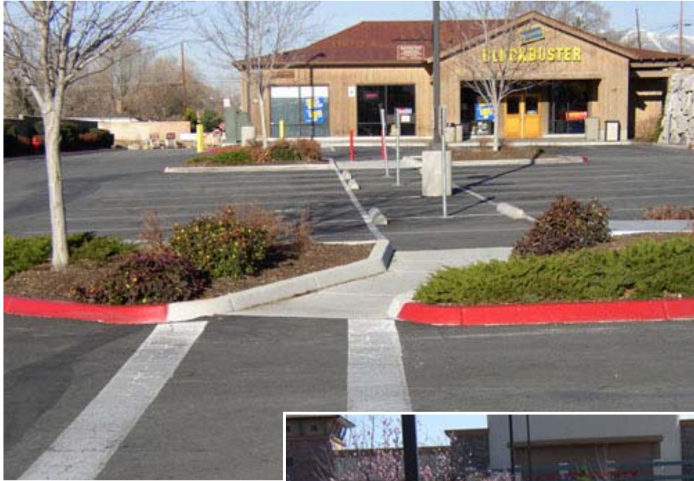
Photo A-2: Pedestrian Walkways within Parking Lots
