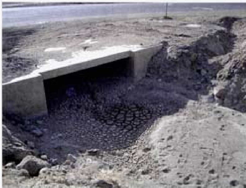
Sediment accumulation in the 12-foot by 4-foot RCB culvert under Toll Road near the intersection with Geiger Grade.
