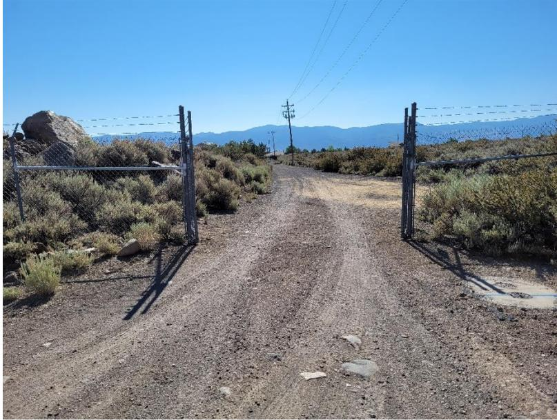
**Figure 5. Existing Perimeter Chain Link Fence**
