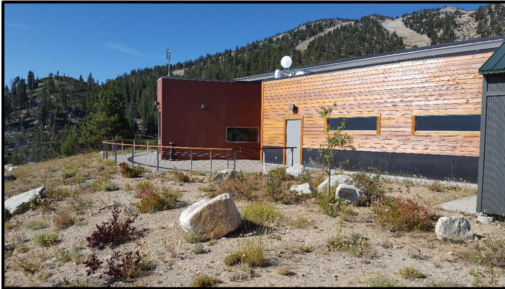
View of the rear (east side) of Winters Creek Lodge – Existing bar area that will be expanded to the southeast can be seen in the projection out from the main building.
