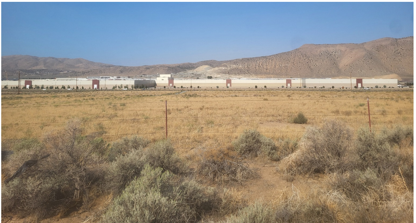
Figure 3D – Site Photo (facing highway from east edge of site)
