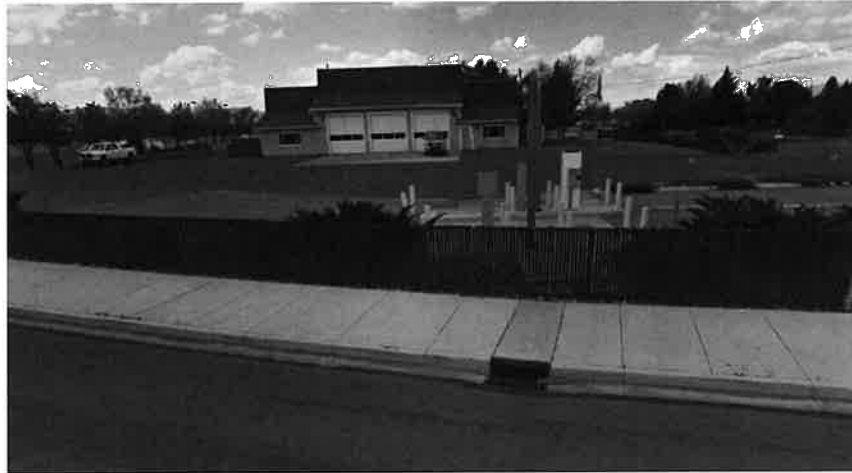
Existing 3-foot fencing along La Posada Drive.
