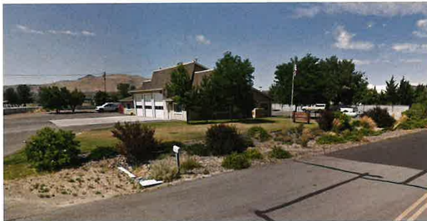
Existing Fire Station #46
