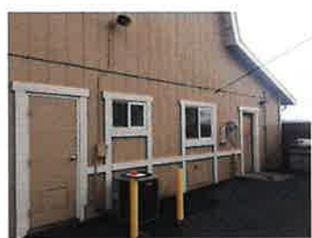
(B4) Existing West Elevation Photo 1 1/2" = 1'-0"
