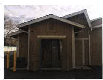
(A2) Existing West Elevation Photo 1 1/2" = 1'-0"
