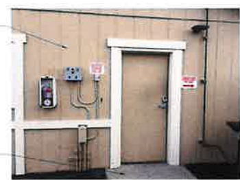
(B2) Existing West Elevation Photo 1 1/2" = 1'-0"
