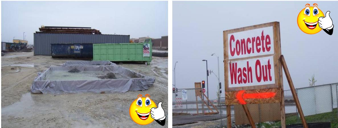
**Figure IC-8c.** The photographs above demonstrate good storm water management practices at a construction site. A dedicated signed concrete washout area is provided in waterproof containment system and the waste materials are recycled (Source: Kennedy/Jenks).
