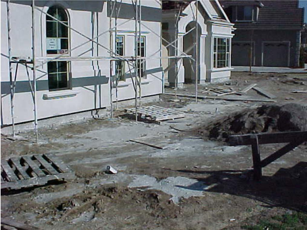
**Figure SC-6b.** The photograph above demonstrates poor storm water management practices at a construction site. Stucco and concrete wastes at this site have been allowed to accumulate on the ground and could become pollutants in storm water runoff. (Source: Concrete Washout Systems, Inc.).
