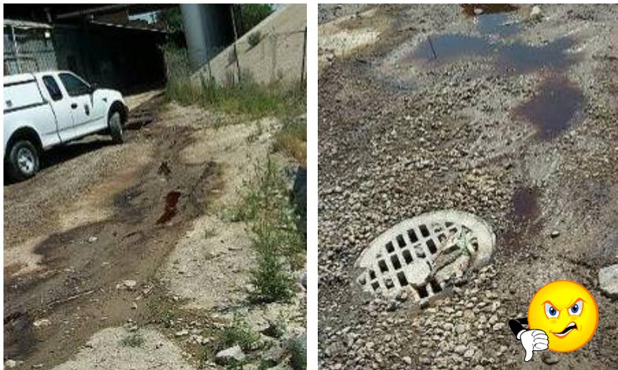
**Figure IC-2b.** The photographs above show a heating oil spill from a local fueling station that was allowed to drain into a nearby storm drain inlet on the right. This is an illegal discharge that resulted in fines. (Source: Reno Environmental Control)
