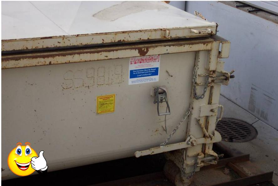
**Figure IC-9a.** The photograph above demonstrates good storm water management practices at a mineral testing laboratory. This hazardous waste dumpster is appropriately covered to prevent storm water from entering and reacting with the contents. The adjacent drop inlet has also been fitted with a catch basin insert (Source: Sparks Environmental Control).
