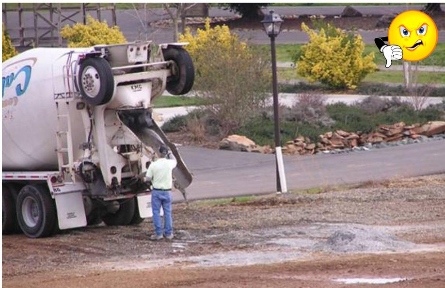
**Figure IC-8b.** The photograph above demonstrates poor storm water management practices at a construction site by a mobile concrete ready-mix operation. Concrete washout should **never** be discharged onto the ground surface, into landscaped areas or into the storm drain system (Source: Concrete Washout Systems, Inc.).
