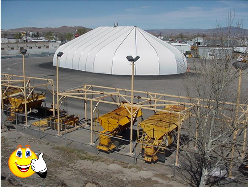
**Figure SC-4a.** The photograph above demonstrates good storm water management practices at a local industrial storage area and maintenance facility. Sand and salt stockpiles are being stored under a sprung tent structure to prevent their exposure to storm water. (Source: Kennedy/Jenks Consultants)
