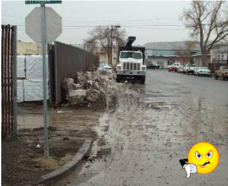
**Figure SC-1b.** The photograph above demonstrates poor storm water management practices. The entrance/exit at this facility has track-out of sediment from a dirt lot onto paved roadways. The sediment and associated pollutants from the site are discharging to the storm drain system, which could result in fines (Source: Sparks Environmental Control).
