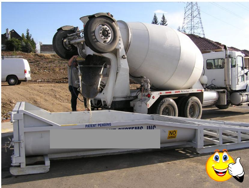
**Figure IC-8d.** The photograph above demonstrates good storm water management practices at a construction site. Concrete washout is contained in a portable washout system and the waste materials are recycled (Source: Concrete Washout Systems, Inc.).
