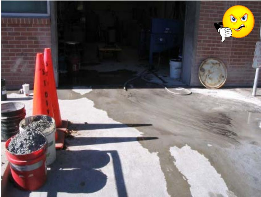
**Figure IC-7a.** The photograph above demonstrates poor storm water management practices - improper containment of stone cutting slurry at this facility has resulted in an illegal discharge to the storm drain system. (Source: City of Reno).
