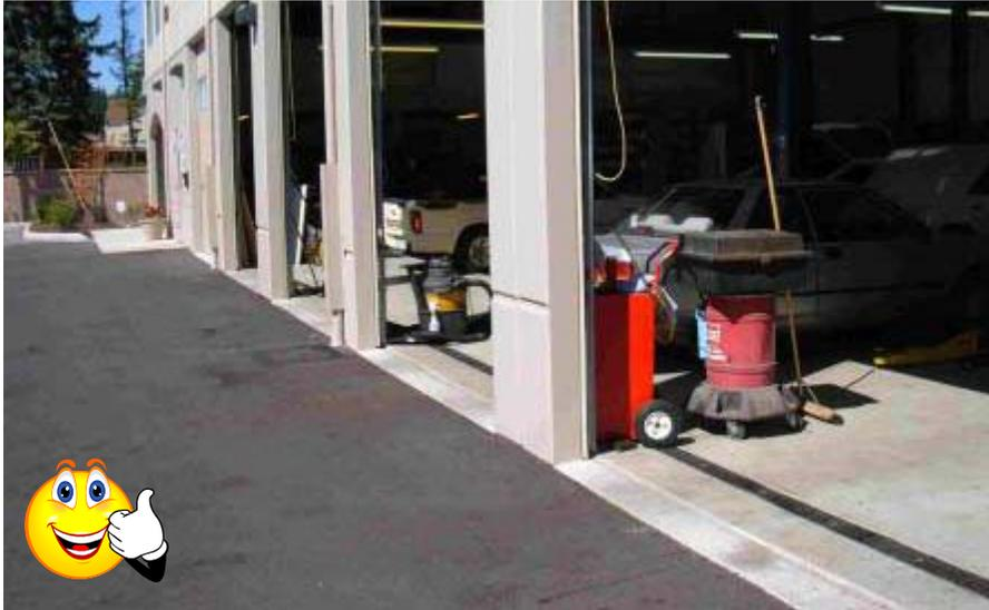
**Figure IC-1d.** The photograph above demonstrates good storm water management practices. A trench drain located near the edge of the covered working area of this vehicle repair facility prevents spills and wash water from draining onto the pavement and entering the storm drain system. (Source: U.S. EPA)
