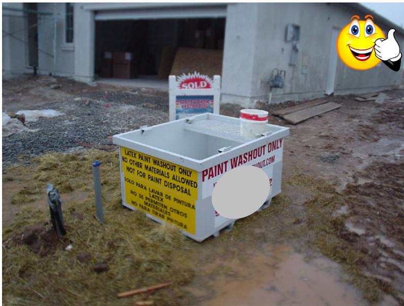
**Figure SC-6b.** The photograph above demonstrates good storm water management practices at a construction site. A dedicated paint washout area is provided in a portable contained system and the waste materials are recycled (Source: Concrete Washout Systems, Inc.).
