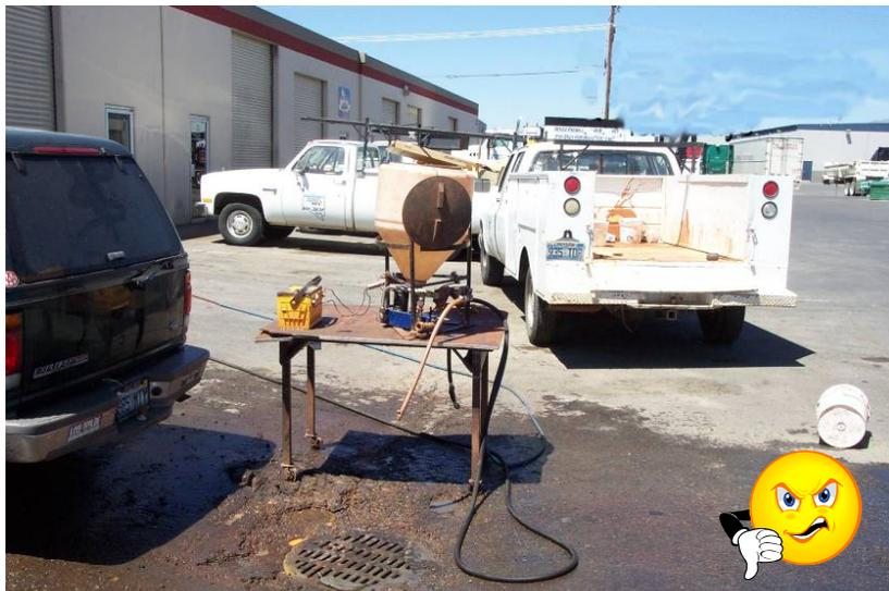
**Figure IC-7b.** The photograph above demonstrates poor storm water management practices - equipment used to dye concrete is being cleaned over the storm drain inlet, discharging chemicals directly to the storm drain system (Source: Sparks Environmental Control).
