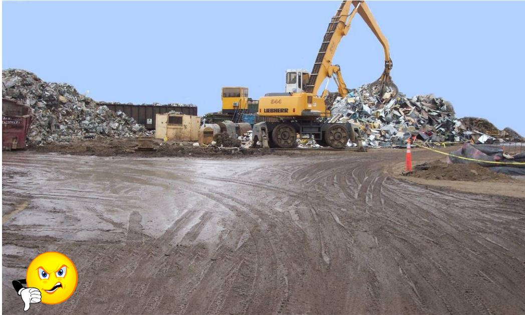
**Figure IC-6.** The photograph above demonstrates poor storm water management practices - improper containment of sediment and runoff from stockpiles. Vehicles exiting site will track out sediment and other pollutants onto paved roadways, which will eventually discharge to the storm drain system. (Source: Sparks Environmental Control).
