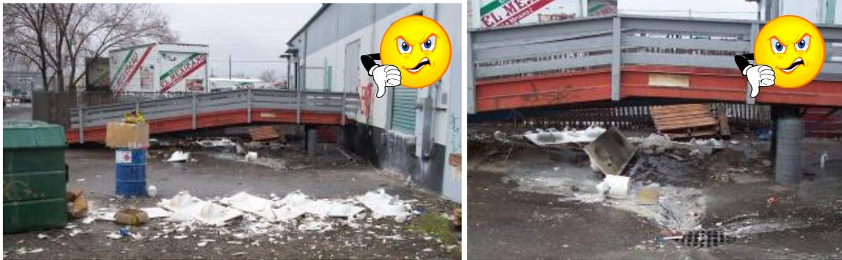
**Figure SC-3b.** The photographs above demonstrate poor storm water management practices – the trash and debris at this loading dock have resulted in illegal discharges to the storm drain system and fines. (Source: Sparks Environmental Control)
