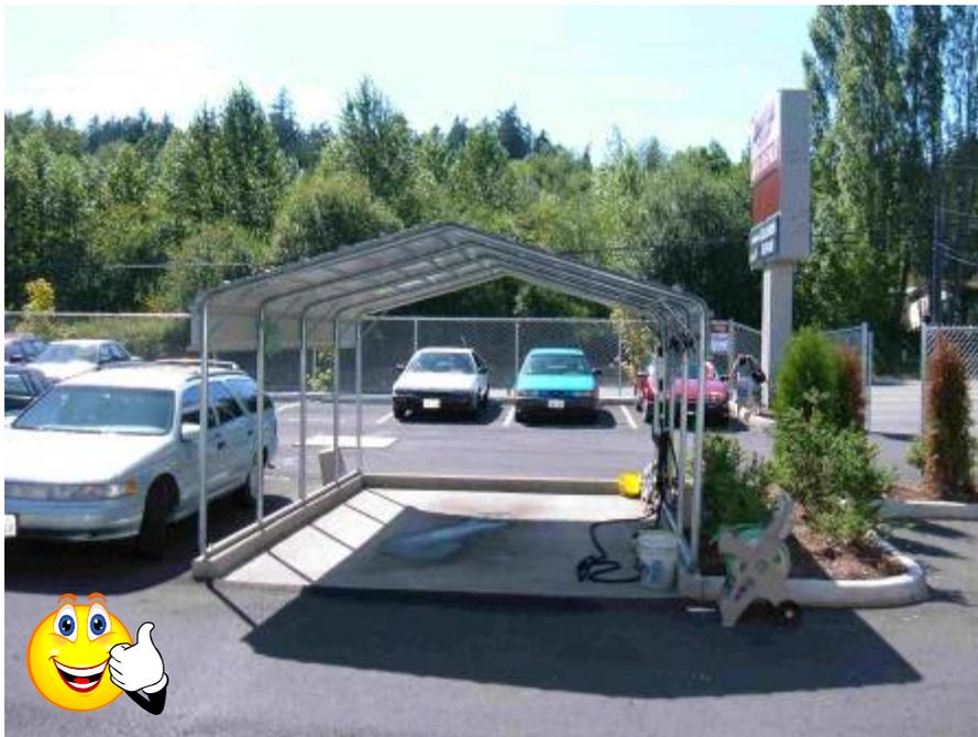
**Figure IC-4b.** The photograph above demonstrates good storm water management practices. A dedicated car wash area at a vehicle repair facility is covered, bermed and graded to drain through an approved pre-treatment device connected to the sanitary sewer. (Source: U.S. EPA)
