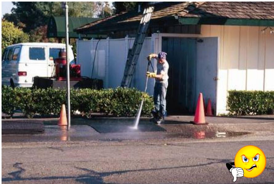
**Figure IC-16b.** The photograph above demonstrates a poor storm water management practice. This mobile power washing operation is cleaning restaurant kitchen floor mats on a public sidewalk. The wash water is being allowed to drain directly into the street and a nearby storm drain inlet. This activity is an illegal discharge to the storm drain system that may result in fines. (Source: CASQA).
