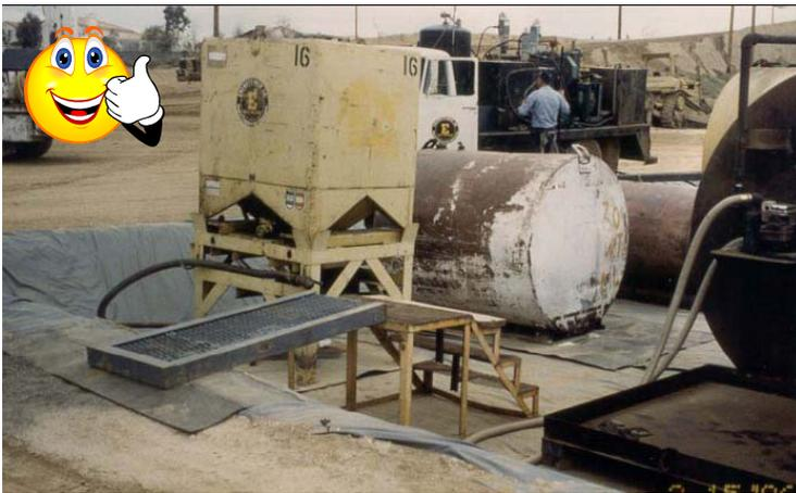
**Figure IC-14a.** The photograph above demonstrates good storm water management practices. Portable fuel and lubrication tanks are temporarily stored in a bermed and lined pit to prevent storm water drainage into the fueling area, to contain any spills, and prevent runoff to the storm drain system. (Source: U.S. EPA).
