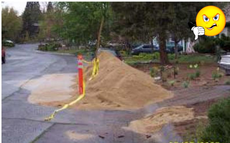
**Figure SC-5b.** The photographs above demonstrate poor management practices. Landscaping materials have been stockpiled on a local street during a rainy period and sediment is being washed into the storm drain system. (Source: Kennedy/Jenks Consultants).
