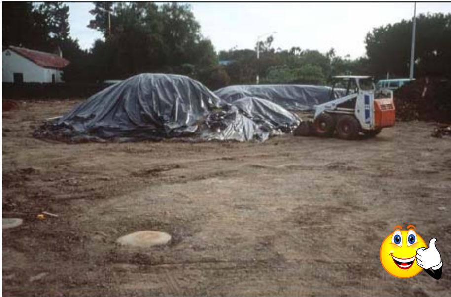
**Figure SC-6a.** The photograph above demonstrates good storm water management practices at a construction site. Temporary soil stockpiles are being covered with plastic sheeting during a rainy period. (Source: CASQA)
