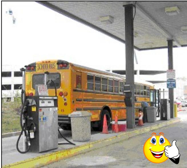
**Figure IC-2a.** The photograph above demonstrates good storm water management practices. This commercial vehicle fueling station is covered and kept clean. (Source: U.S. EPA)
