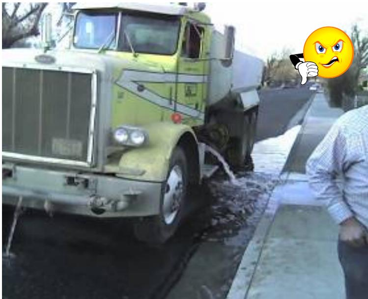
**Figure SC-1c.** The photograph above demonstrates a poor storm water management practice - improper disposal of reclaimed – non potable water for dust control. This practice is an illegal discharge that could result in fines. (Source: Reno Environmental Control)
