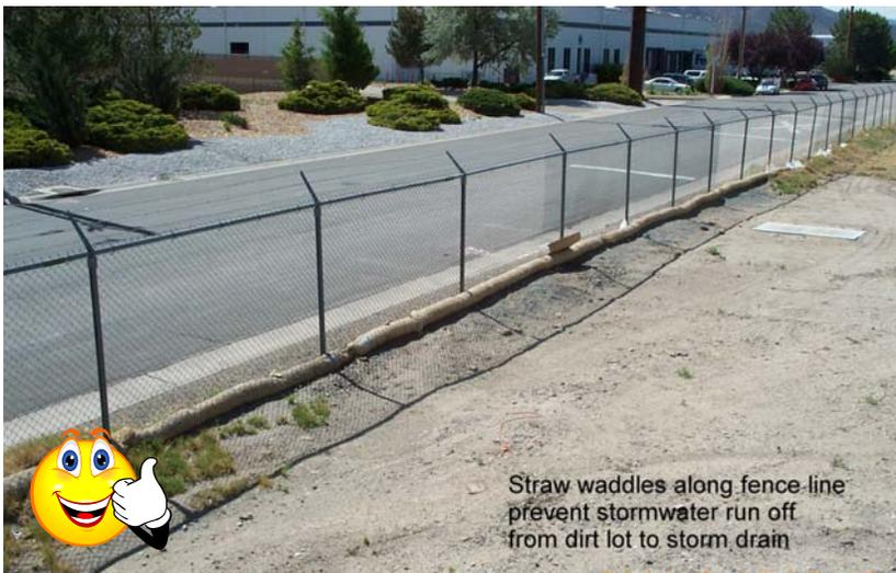
**Figure SC-4b.** The photograph above demonstrates good storm water management practices at a local industrial storage area. Fiber rolls or straw waddles have been placed along the perimeter of this dirt lot to prevent sediment and associated pollutants from being washed off the site and into the storm drain system. (Source: Sparks Environmental Control)
