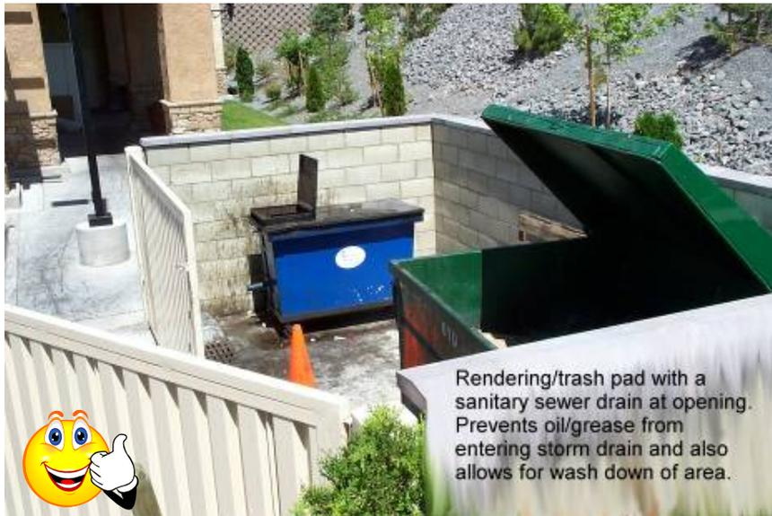
**Figure IC-10a.** The photograph above demonstrates good management practices at a local restaurant. The trash enclosure is kept clean and drains to the sanitary sewer system (Source: Sparks Environmental Control).
