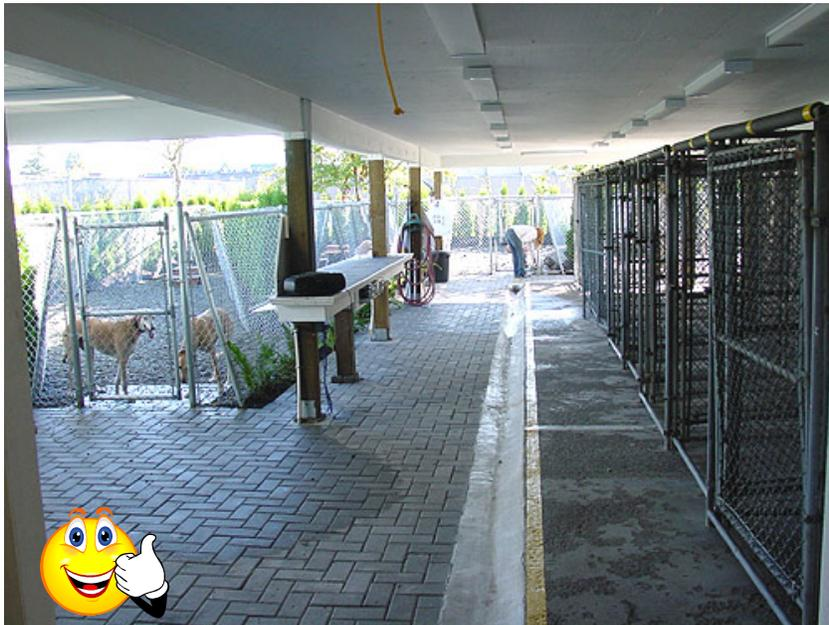
**Figure IC-11b.** The photograph above demonstrates good storm water management practices. Animals at this handling facility are kept in areas that can be easily cleaned and maintained. Wash water is channeled into a drain connected to the sanitary sewer system (Source: Rondivills Kennels).
