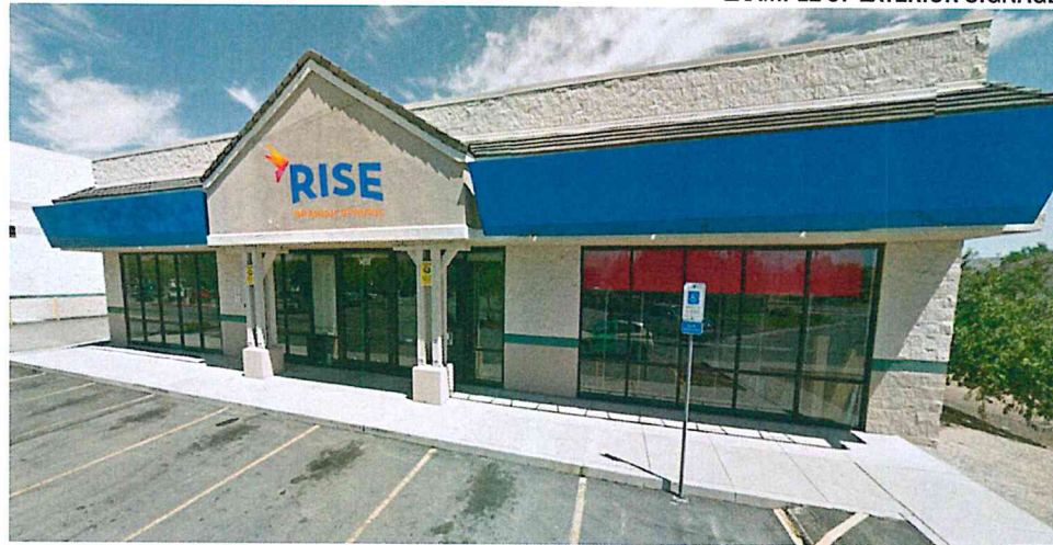
EXAMPLE OF EXTERIOR SIGNAGE
