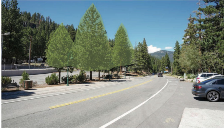
EXISTING SITE CONDITIONS
