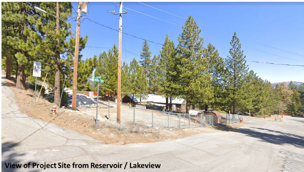
View of Project Site from Reservoir / Lakeview
