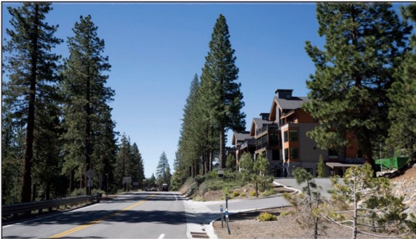
EXISTING SITE CONDITIONS
